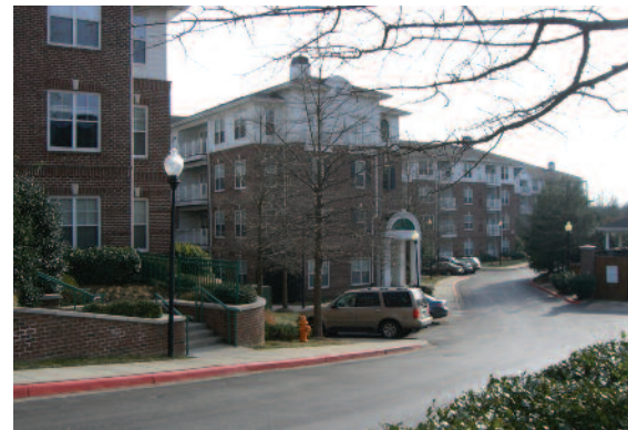
Far Left: Office uses may be appropriate on Parcels I and L. At Left: Multi-family development could be considered for Parcels L and M.
